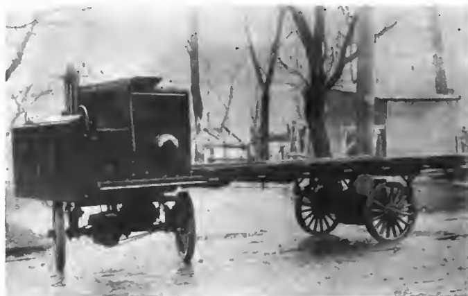
NEW GASOLINE-ELECTRIC TRUCK FOR HEAVY WORK.
